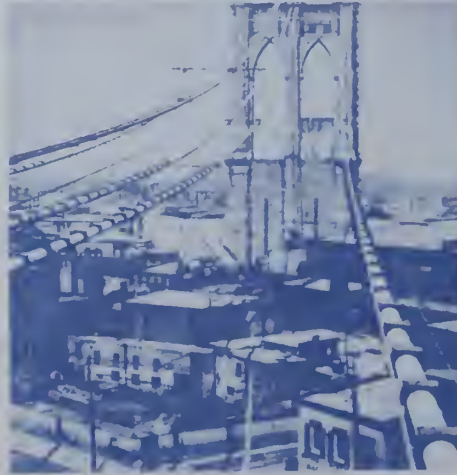
These views of the bridge about 1879 show the completed cables.
